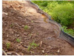
Silt fence, properly installed, keeps sediment from washing into streams. It also prevents the need to install it a second time, saving you time and money. The sediment will need to be removed from this fence to keep it functioning.
