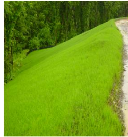
Proper and timely site stabilization prevents erosion, protecting streams and saving you time and money. Stabilization of this slope will prevent erosion.
